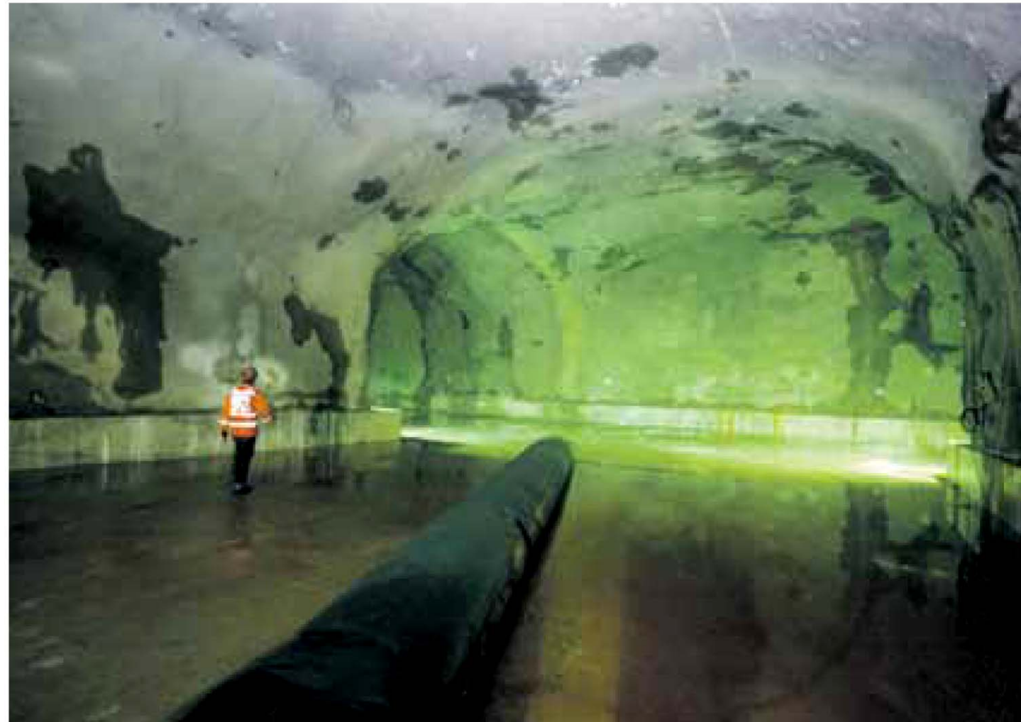
The underground rock cavern oil storage project at Jurong Island. Underground caverns may soon be used to expand Singapore’s water storage capacity and alleviate flooding. PHOTO COURTESY JTC
